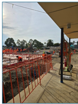
North facing from the Hall
