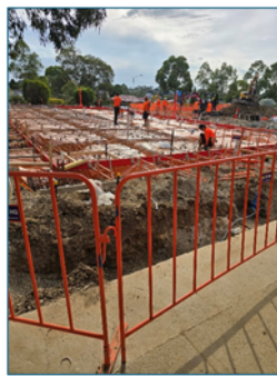
The Administration Building
