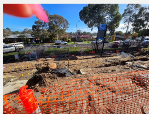
Beginnings of a ramp
